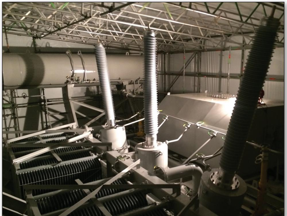
*The first of the Paraparaumu transformers enclosed in the wrapped scaffolding.*
